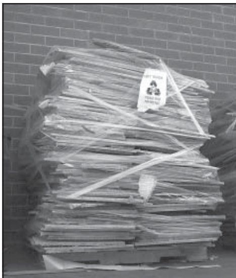
Ceiling tiles awaiting pickup for recycling.
