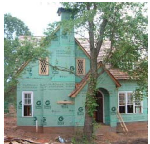
New construction at Hedgewood's new EarthCraft Vickery development
