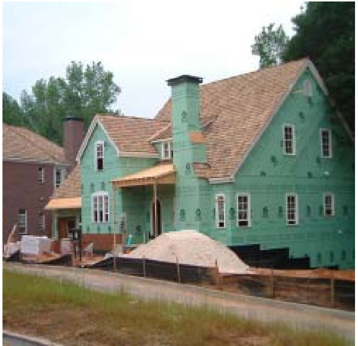
Scrap drywall has been ground for later land application onsite at one of Hedgewood's EarthCraft construction sites. Scrap drywall diverted from the landfill can be a valuable soil amendment when properly applied.
